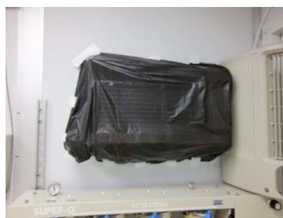
Figure 3: Preparing an AC unit to be replaced by covering it with plastic prevents outside particles from entering the cleanroom
