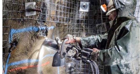
Figure 7: Infrastructure Tech Talon Tucker uses a chainsaw to cut or "gad" rock in the Ross Shaft
