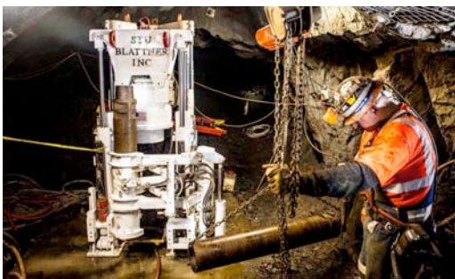
Figure 5: A crew from Stu Blattner Inc. changes a pipe on a drilling rig at the 1700 Level. The cylinder in the foreground is a button bit cutter. The reamer uses four of these cutters and is pulled up or back reamed to widen the pilot drill hole, creating a raise.
