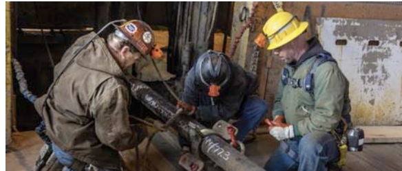
Figure 6: Rope Technician Rick Tinnell and Infrastructure Technicians Jason Graves and Pat Urbaniak prep a 33-foot pump motor to be lowered down to the Yates Shaft
