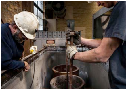
Figure 5: Facilities Technicians Kevin Ehnes and Chris Huber install electrodes into the clay pots in the slip regulator tank
