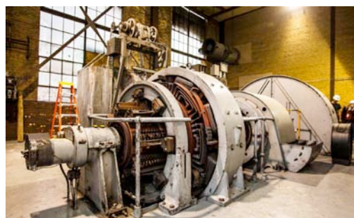
Figure 4: The motor-generator set that converts AC power to DC power to operate the hoist.
