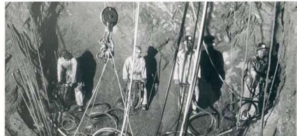
Figure 8: Deepening the Yates Shaft, 1954: When the pilot raise was completed, stripping crews slashed out the sides of the raise, bringing it to its full dimension of 15x27 feet, eight inches (Photo Courtesy of Homestake Mining Company and Stephen Mitchell)
